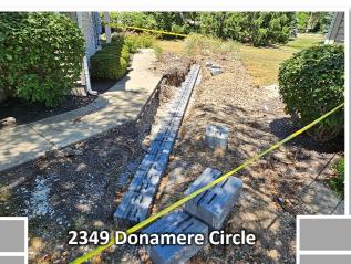
season. The original railroad tie walls are being removed, and then being replaced by cement Versa Block walls.
